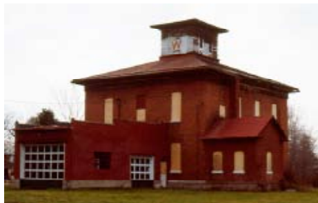
4th Ward School, Washington Street, early 1980's vacant and deteriorating
