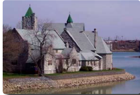
Trinity Episcopal Church, 2006 - lowered water level shows effective shoreline preservation treatment
