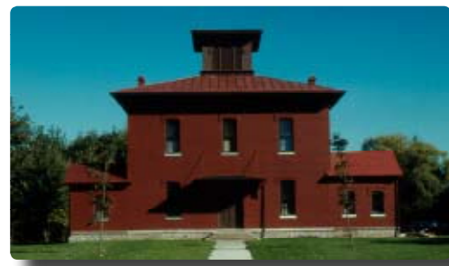
4th Ward School, Washington Street, late 1980's exterior restored, interior converted to four condominiums
