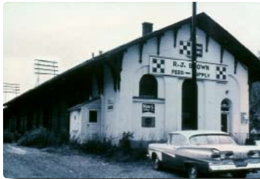
NY Central Freight Station, 1970's vacant feed supply store
