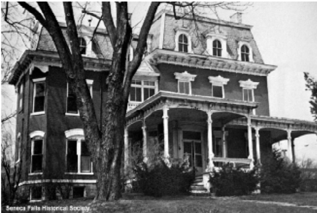
The Armitage - Demolished
